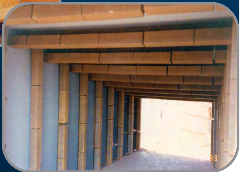
2x2x9 inch Vidablocks fitted into a chute that forms part of a fines reduction plant at an iron ore port.
