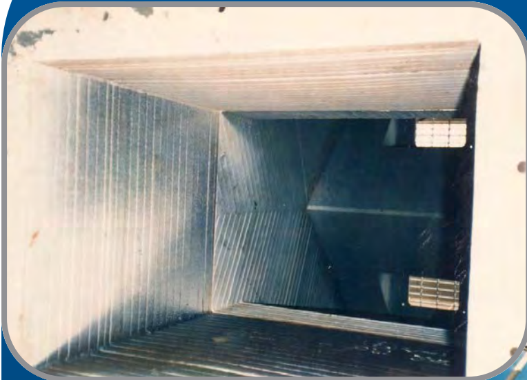
Fabricated Vidaplate chutes.
